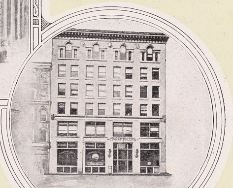
Boston Office 126 State Street
