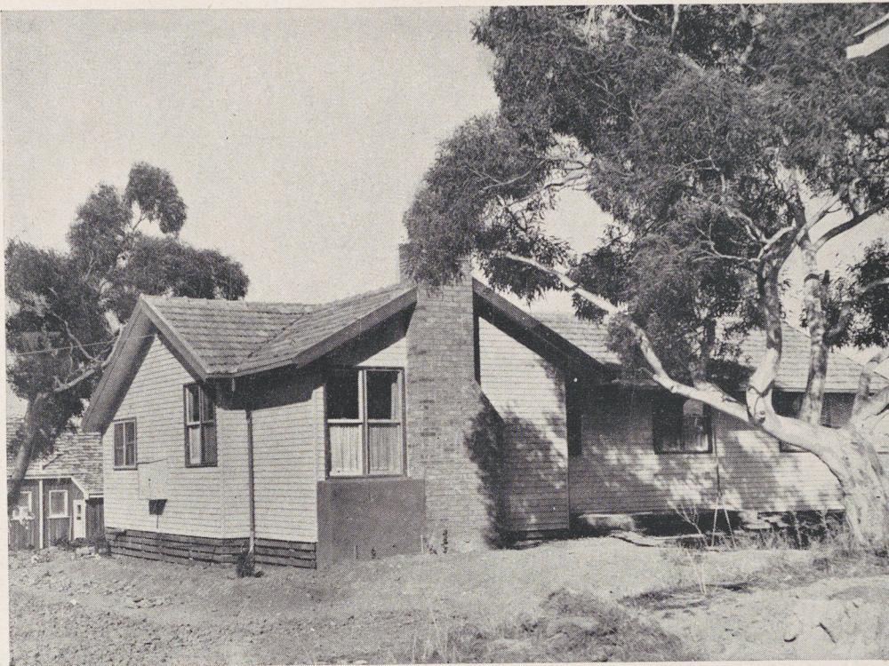
One of the Authority's staff houses in the Headquarters Township, Cooma North, built by an Italian contractor.
