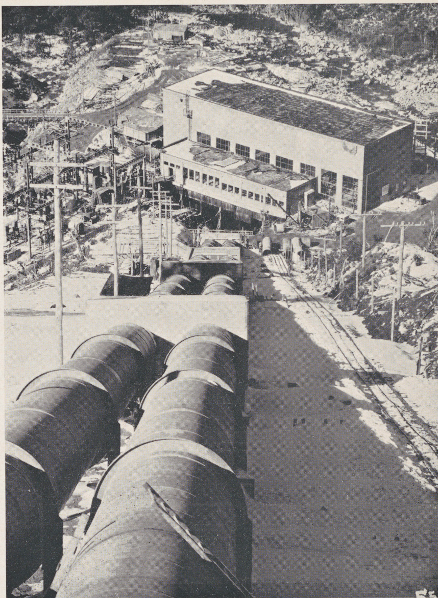
Guthega Power Station during construction in winter of 1954
