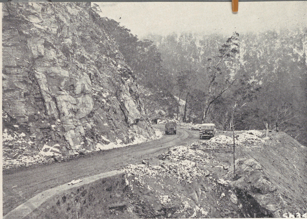
Road constructed by the Authority in the Tumut River Gorge between Cabramurra and T.I Power Station site.
