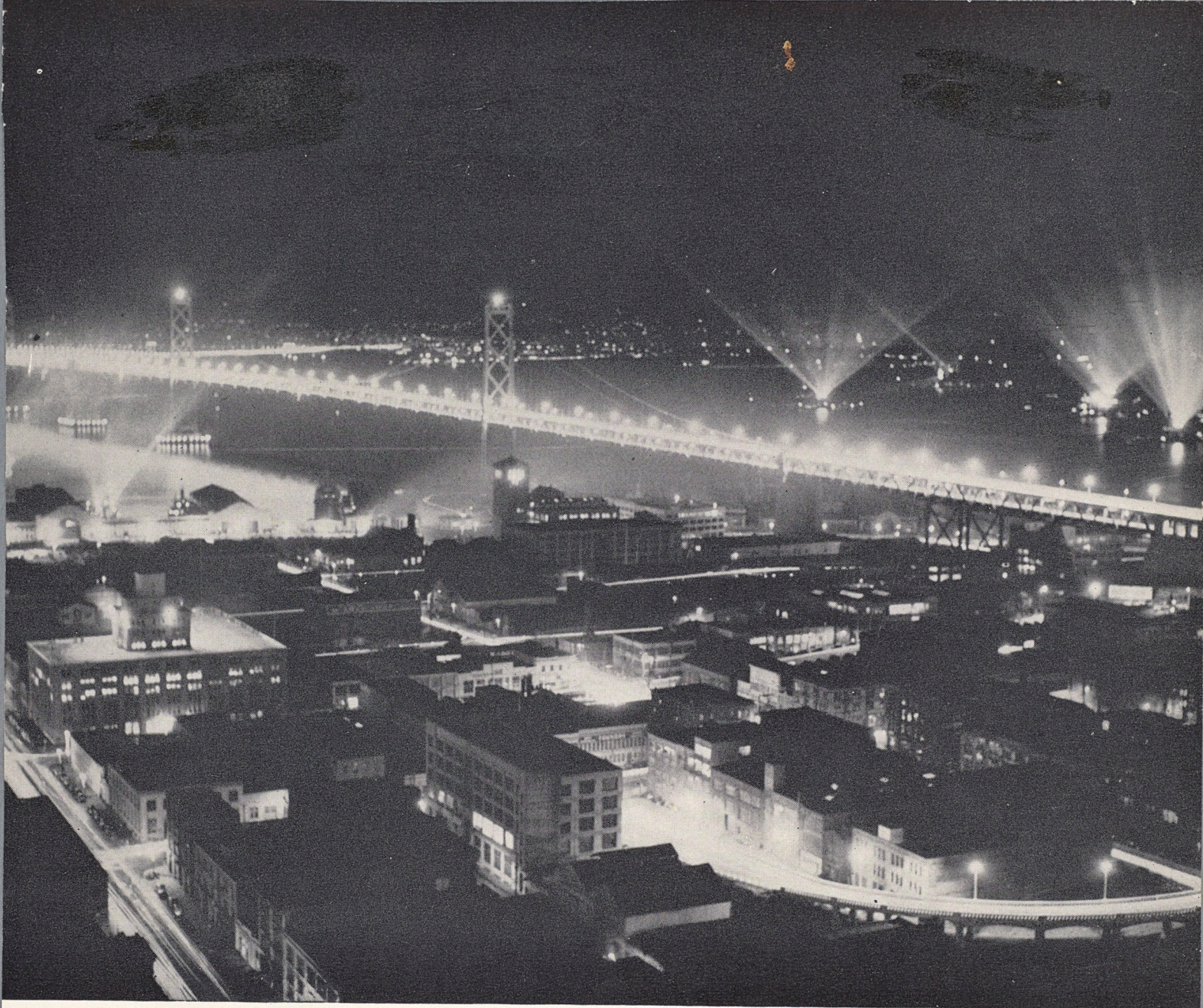
Like a chain of pearls, the San Francisco-Oakland Bridge sparkles over the Bay.
